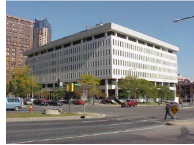
Warren E. Burger Federal Building and U.S. Courthouse
